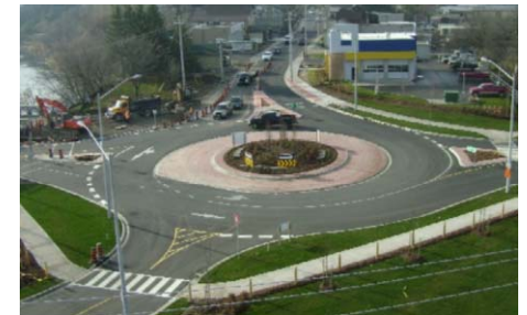
The Region of Waterloo considers roundabouts at every intersection where signals warranted
